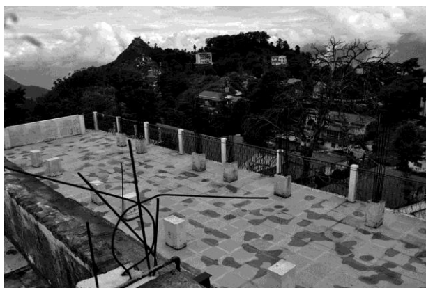
The proposed place of installation for the solar water heaters; located at the heart of the campus where the sunlight is direct
