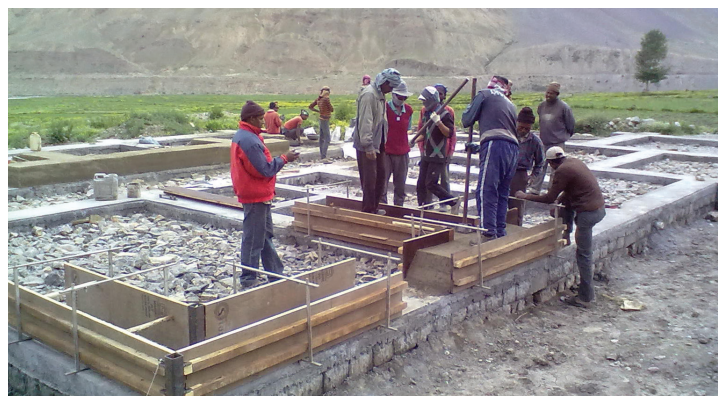
Photos - Top: Completed first floor of the Community Centre Bottom: Building work using rammed earth technique
